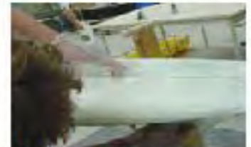
(h) Overhanging wet cloth was lapped with squeegee underneath
