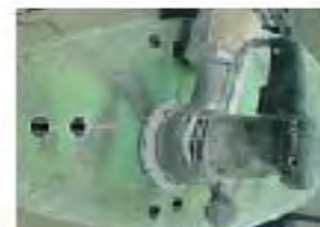
(q) The excess resin was removed and the surface smoothed.
