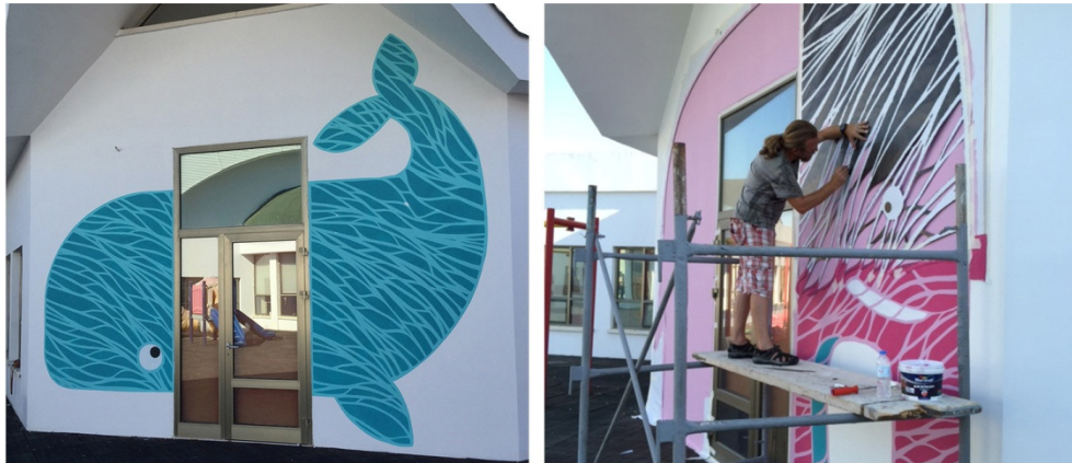
Figure 6. Stencil Works for Near East Nursery Playground Doors
